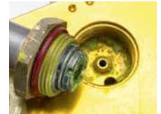
Sealant contamination in the A/C service unit without the use of the Recycle Guard
